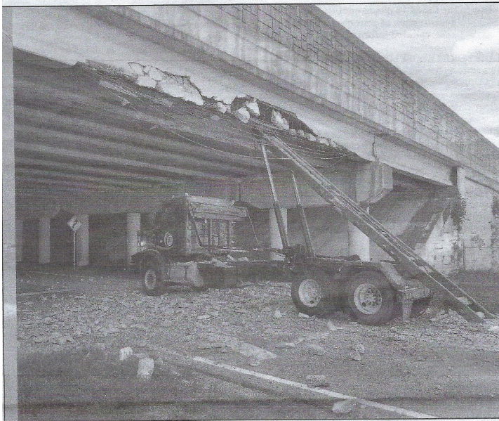
Sudden Stop! A City of Lake Worth Beach roll off dumpster truck struck the I-95 overpass at 12th Avenue South Tuesday weakening the structure of the overpass. Below: On Wednesday, crews from Florida Department of Transportation and The City of Lake Worth Beach gather to assess the damage.
